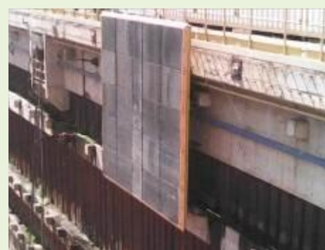
DEFENSER DE PLACA METALICA C/ BAQUELITE E BORRACHA DO DIQUE DIM 6,10X6,10 M | Item: 200086 |
