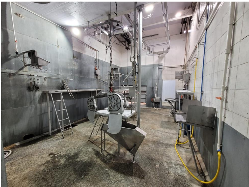
Interior Galpão Principal
