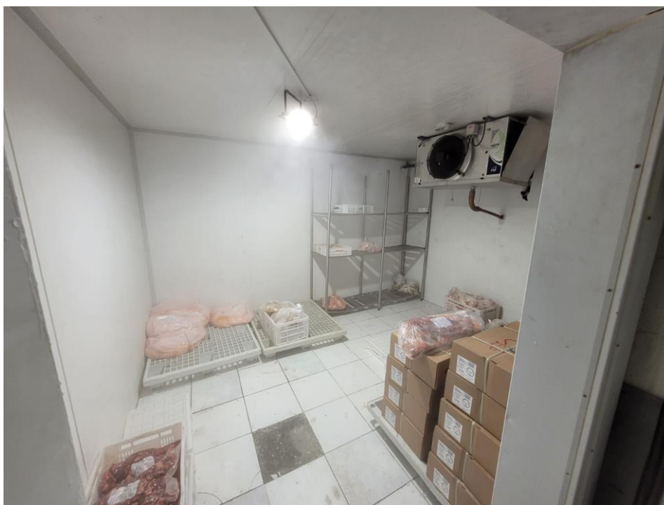
Interior Galpão Principal
